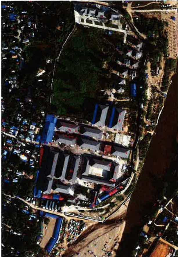
Fig. 8 – Analysis of Starlink Terminals (circled in red) at Shunda Compound.
